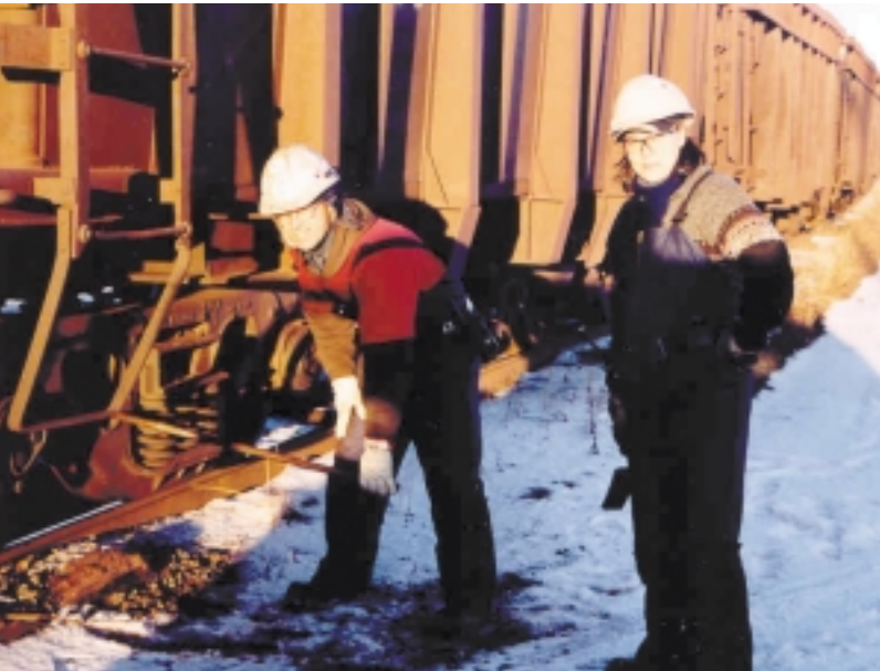
Marcel Marticotte and Guylaine Pigeon (Maintainers/Operators Mechanical 2) replace the brake shoes on the cars.
